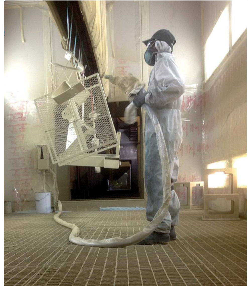
Second anti-corrosion coat and top coat
